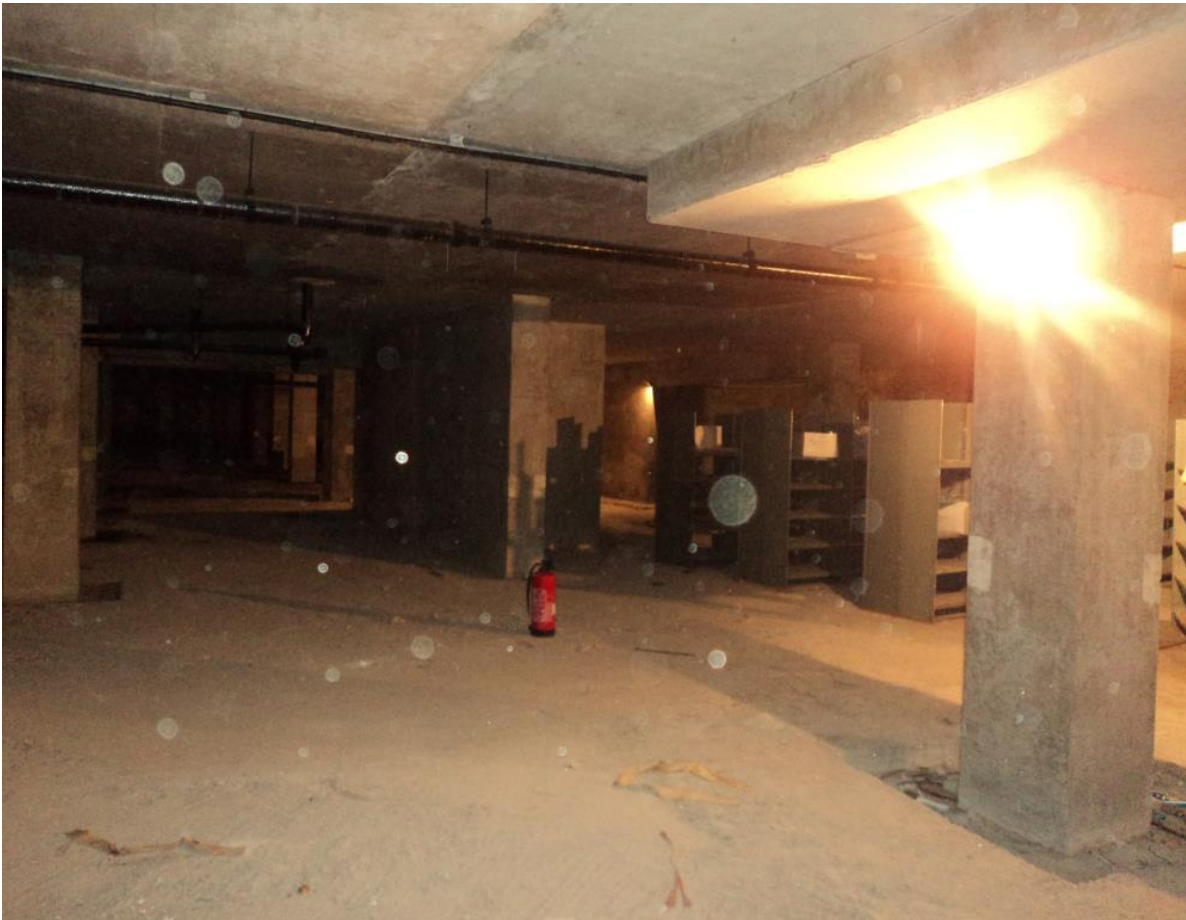
Internal view of existing grade II listed vaults
