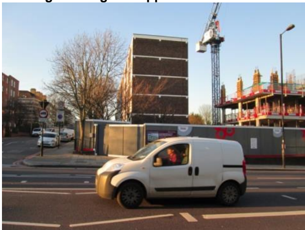
John Barnes Library site (under construction)
